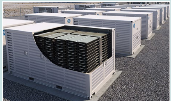
Representative view of a storage facility.
